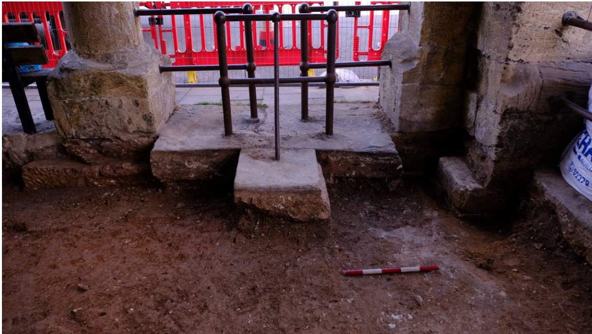
Fig. 19 View of north-western corner showing original foundations, threshold slabs and iron baffle gate; scale 0.5m
