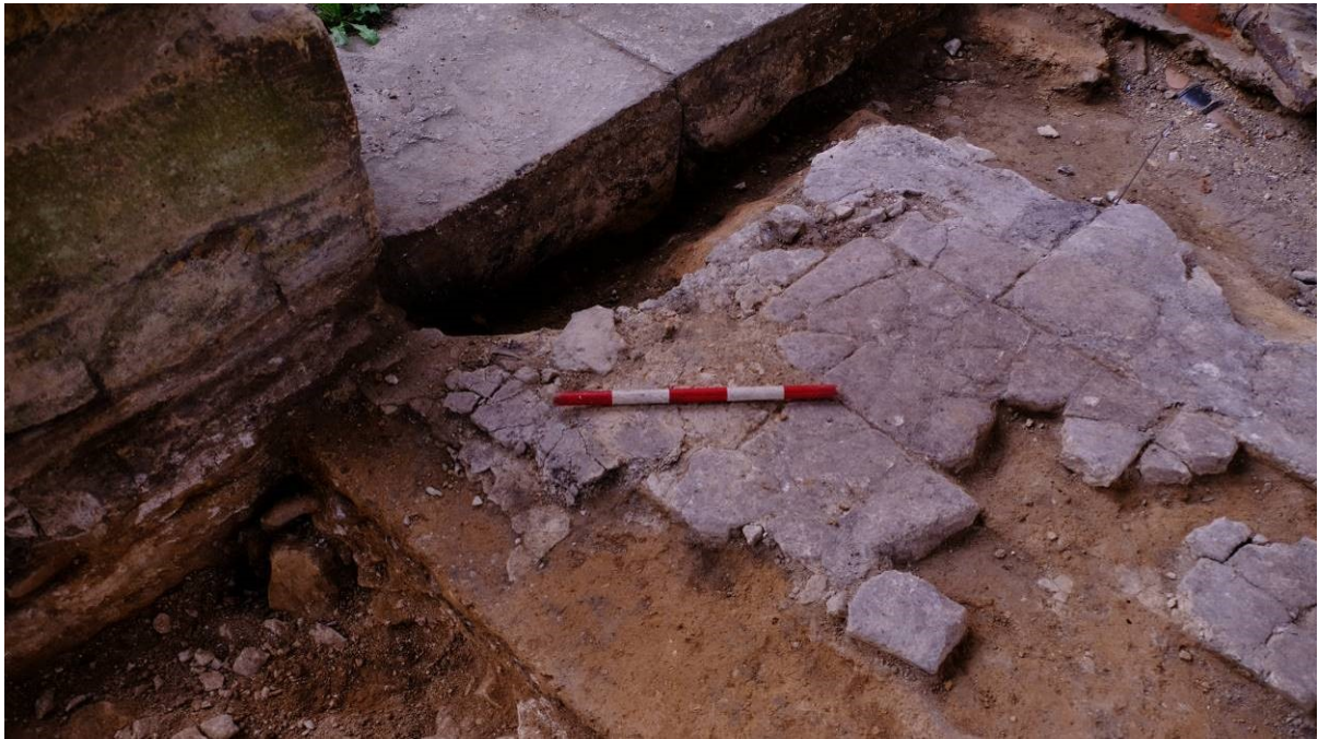
Fig. 17 View of paver floor [46] on clay slab (47) truncated by cut [44] for threshold slabs. Note the pavers are beneath the base of the pier superstructure, and the clay slab abutting the foundation; looking south, scale 0.5m
